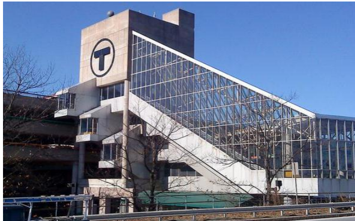
Figure 1: Image of Alewife MBTA Parking Garage Station Complex from a Street View [1]
